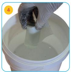
Wearing the enclosed gloves remove the Repair Wrap from the foil pouch and soak the roll in temperate water for 20 seconds.
