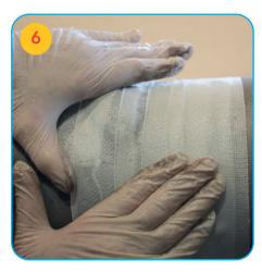
Squeeze and mould Repair Wrap in the direction of the wrap, removing excess water and spreading resin until it is tacky to touch. Allow 30 minutes for resin to set.
